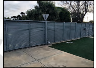
Figure 2. Steel Fence Location and Environment
