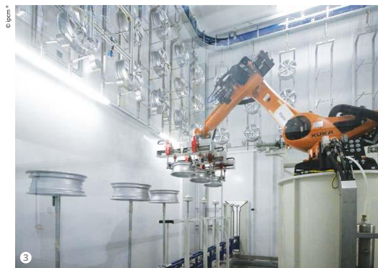
Figure 3: The robotic transfer from the overhead conveyor of the pre-treatment circuit to the floor conveyor of the powder application circuit.
