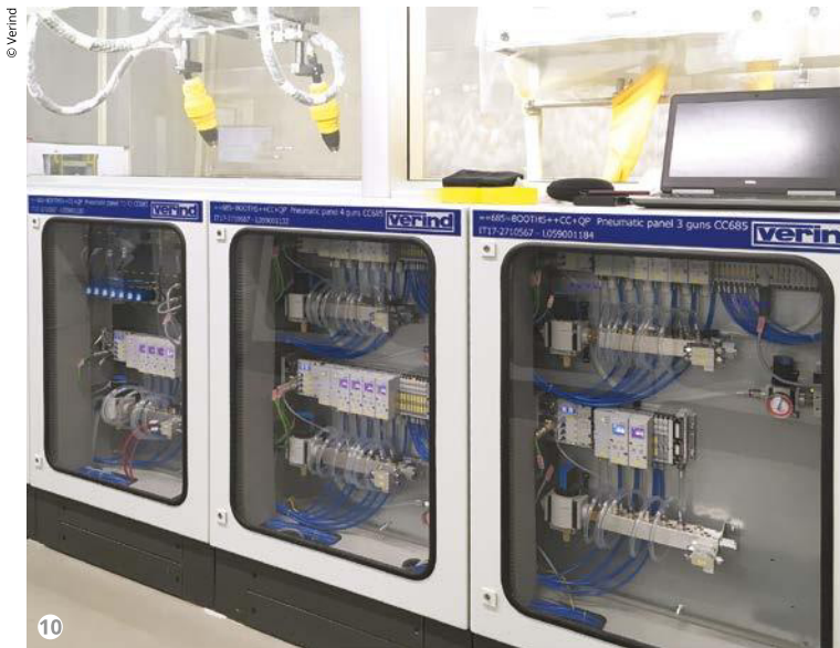
Figure 10: Automatic control panel of paint application parameters of EcoBell and EcoGun.
