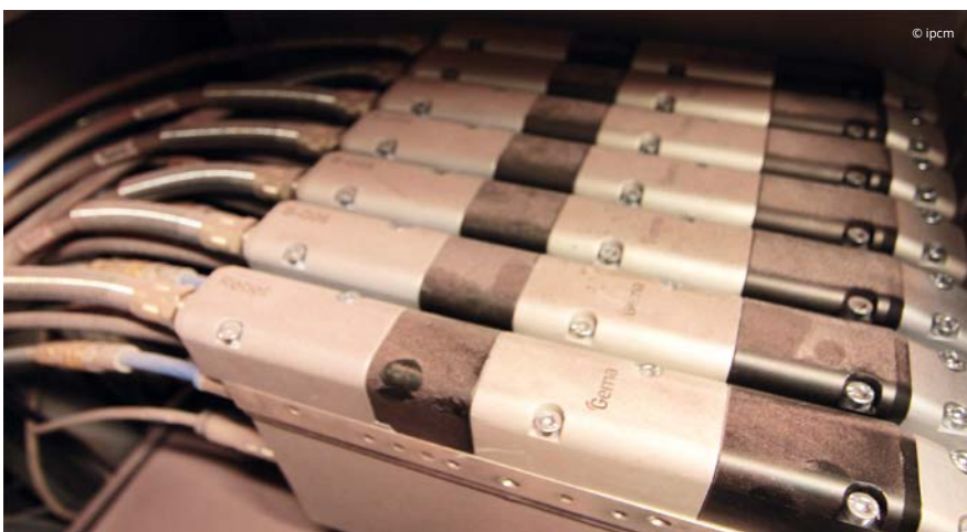
The dense phase pumps.
