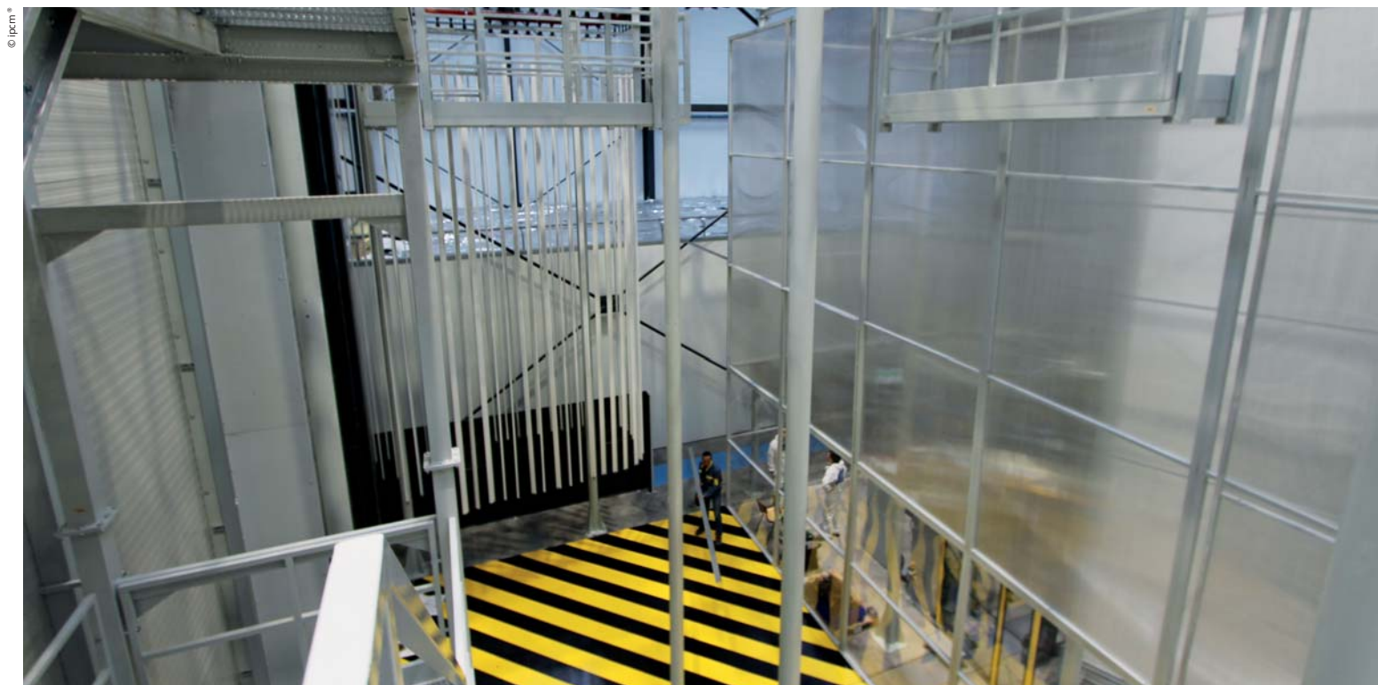
Detail of the vertical coating installations
